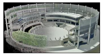
All ducting, piping and cable runs were identified and shown in the model. Underground services were also surveyed and implemented into the MEP model, and a complete as-built BIM-ready model was delivered.
