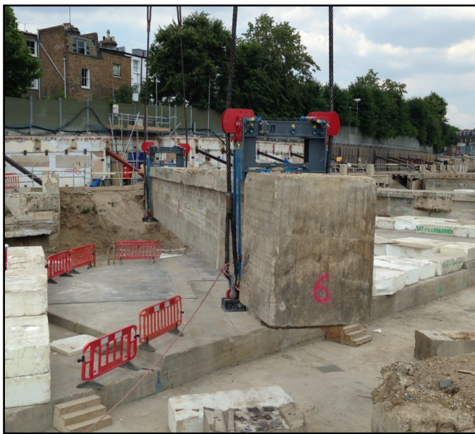
Removing the 62 portal beams
