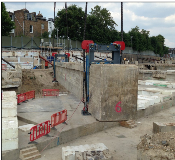
Removing the 62 portal beams
